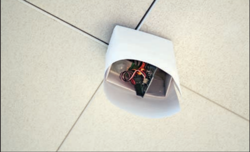
Passive infrared sensors detecting presence.
